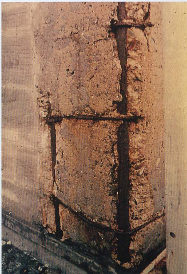
Fig. 1: Corrosion of rebar caused by inadequate concrete cover.
