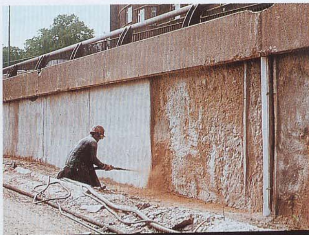
Fig. 2: Renovation of a reinforced support wall.
