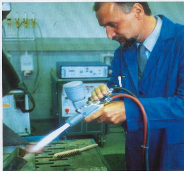
Fig. 5: Repair by thermal spraying with zinc
