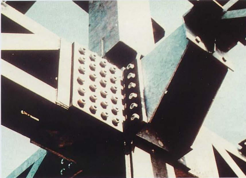
**Fig. 3 : Hot dip galvanized high strength bolts in a bridge structure.**
