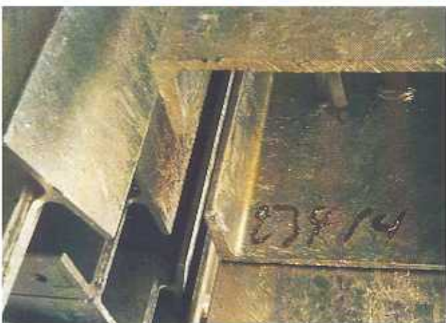
Figure 3: Flaws due to paint markings.
